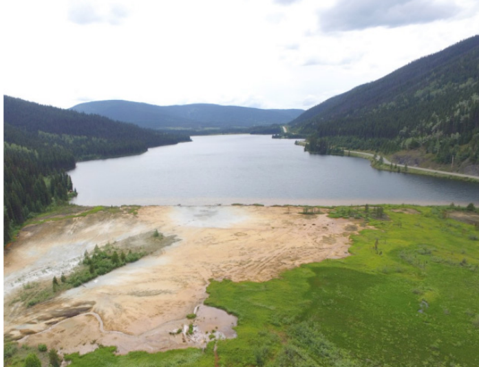
Island Mountain tailings as seen from east to west
