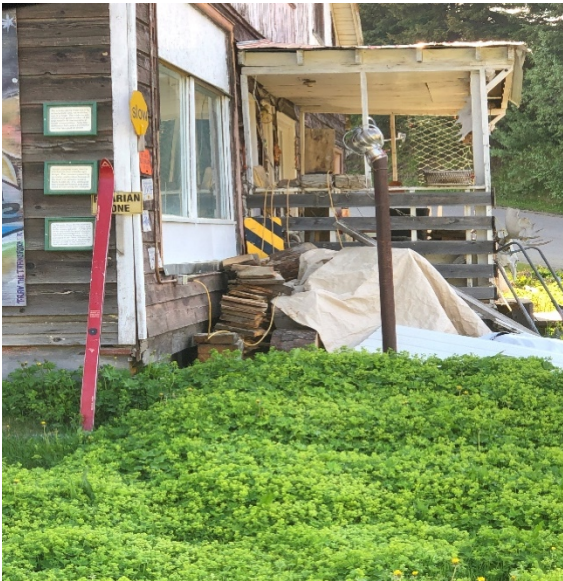
High percentage of structures have firewood stacked next to them. Blowing embers can land in the wood piles, ignite them and then the structure.
