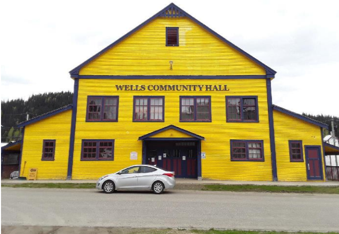
Figure 6: Wells Community Hall – example of critical infrastructure needing FireSmart materials improvements
