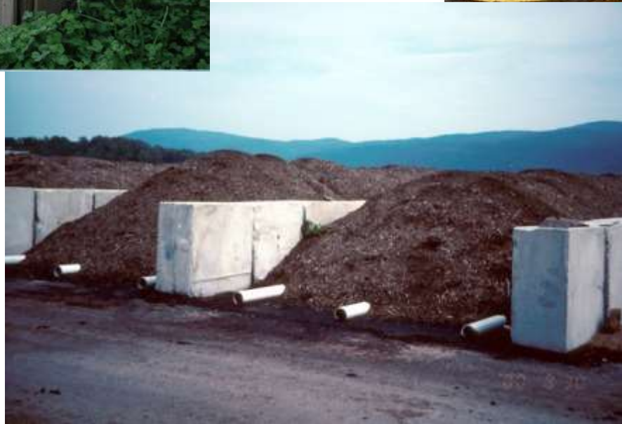
Open windrow with passive aeration (Grand Forks, image Vermont)
