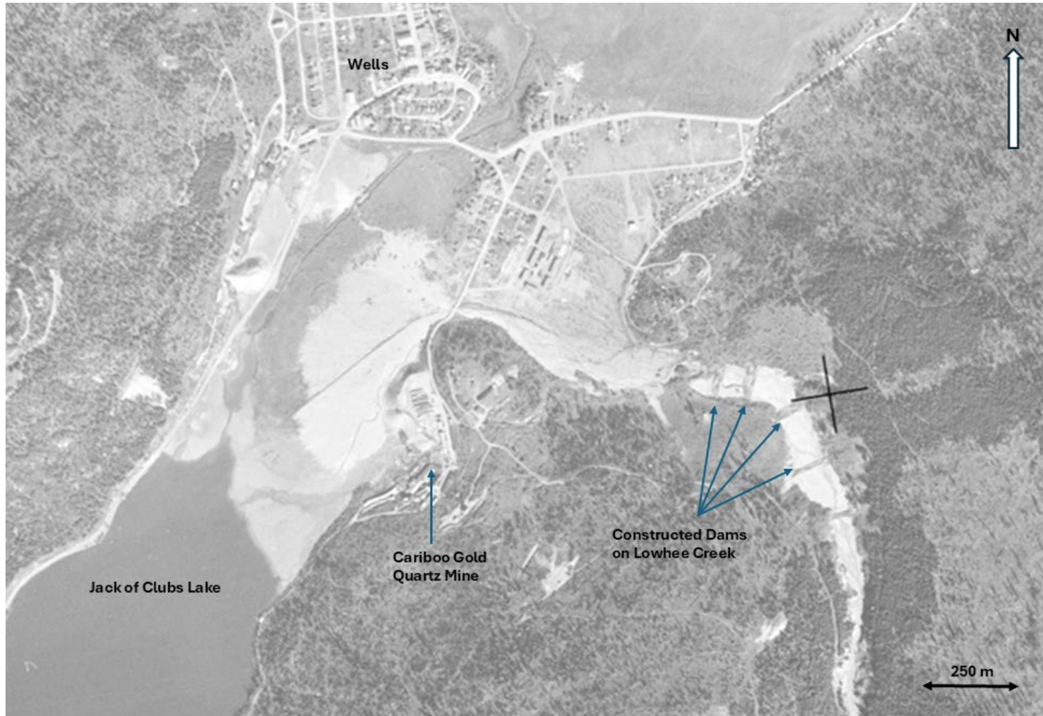
Figure 3-3 1952 airphoto showing constructed dams within the Lowhee Creek lower watershed. Photo source: National Airphoto Library 4 , September 1, 1952.
